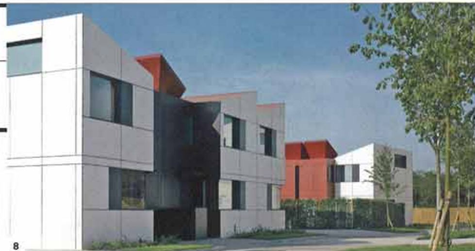
8 Oxley Woods, by Rogers Stirk Harbour + Partners for Taylor Wimpey. Completed in summer 2007 as part of English Partnerships' Design for Manufacture programme; 145 homes over 3ha
